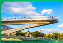
Floating Bridge Moscow
